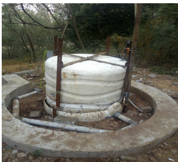
Fig1.4. Main Digester Tank Installed At YCCE
