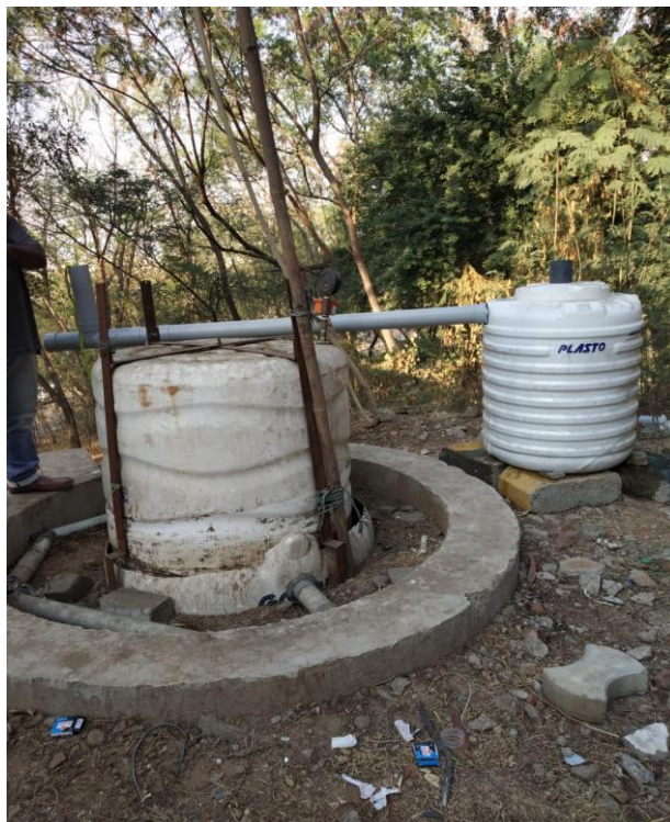
Fig1.5. Overview of the complete Plant
